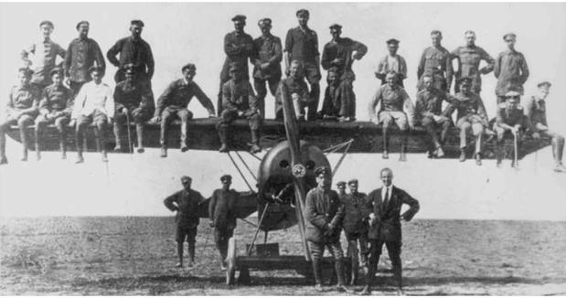
**Fig. 5** Sleek 1918 Fokker D.VIII monoplane foreshadowed a coming standard with its thick-sectioned, plywood-sheathed, cantilevered single wing; Anthony Fokker, in front in necktie, humorously demonstrates the strength of the D.VIII wing design (SI negative number A2185).
